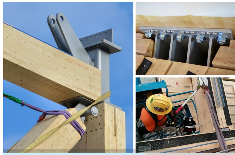
Slotted-in plates with tight fitting dowels
