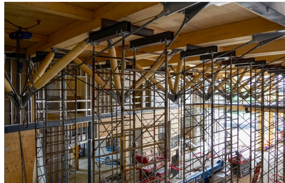
Slotted-in plates with tight fitting dowels
