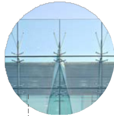
Curtain wall, with rainscreen and metal structure to support open atrium
