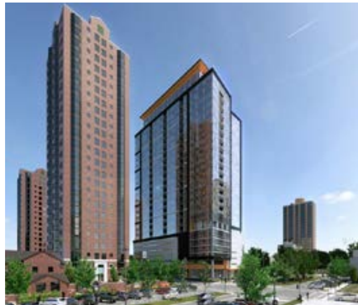
Figure 31: Exterior View Of Ascent MKE, Peronto, 2020
