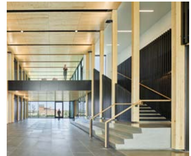
Figure 38: Catalyst Spokane interior atrium featuring Glulam and CLT, Darling, 2020
