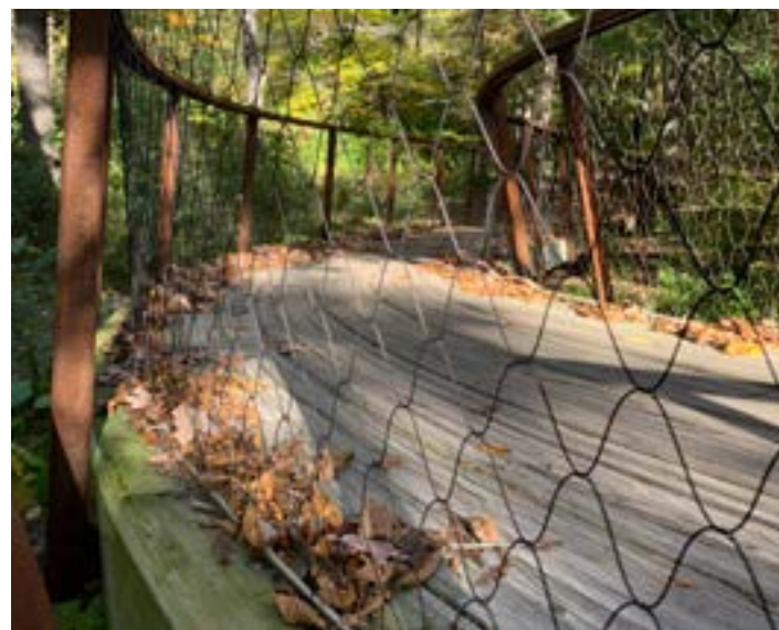
Figure 15: Timber Bridge in Connecticut, Self provided, 2020
