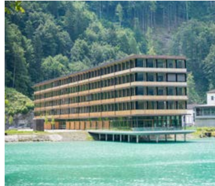
Figure 34: Illwerke Zentrum Montafon exterior view, Pachnicke, 2020
