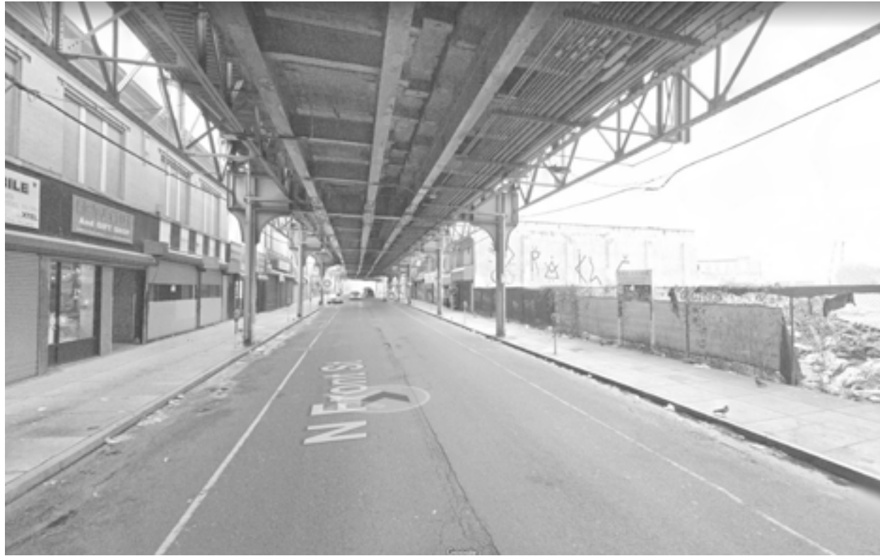
Figure 30. Existing Condition of the "EL"
